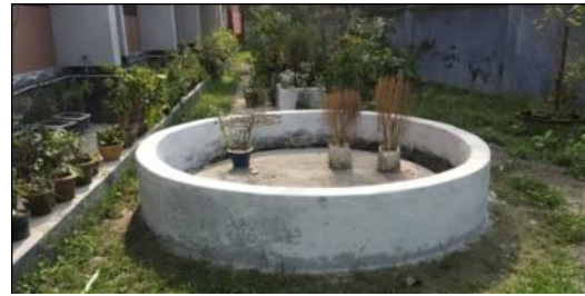
Fig :Septic Tank of BN school and college
